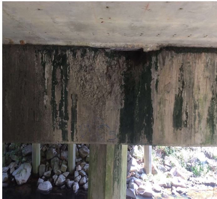
PHOTO 1 Description CONCRETE CAP BT 2 WEST FACE 2'X1.5' SPALL W/REBAR EXPOSED W/SECTION LOSS
