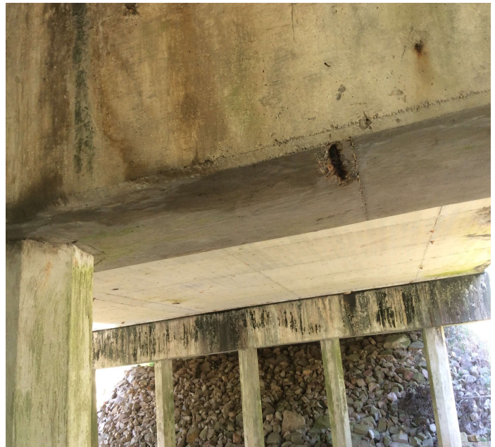
PHOTO 2 Description CONCRETE CAP BT 3 BOTTOM OF CAP MINOR SPALL W/REBAR EXPOSED BETWEEN PILE 1 & 2
